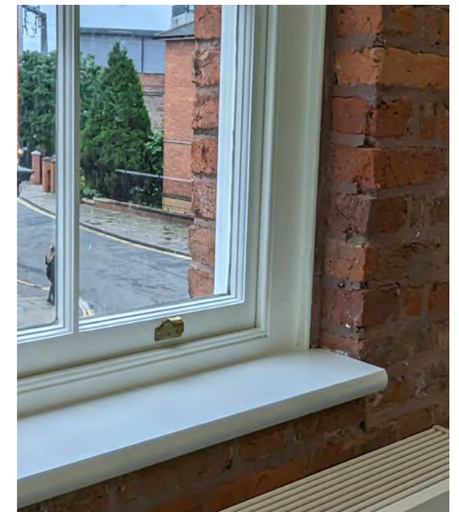
Above: Newly repaired sash window
