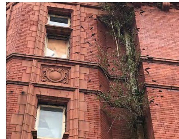
Far Left: Image showing rainwater goods on domestic property.
